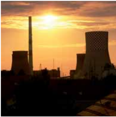
Lagisza Power Plant, Poland
