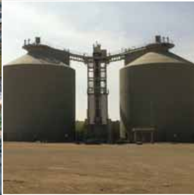
Abu Dhabi WWTPs, UAE
