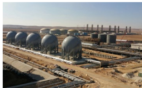
Amman Petroleum Product Terminal, JOR
