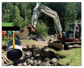
(g) Pipe damage (excavation works), August 2019.
