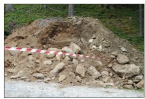
(c) Excavation/ backfilling material of the pipe trench with rocks of up to 1 m in diameter, summer of 2019. 1.5 times the operating pressure would not have been possible for the pipe (potential destruction incident = failure of the pipe) and that therefore this test was not conducted at 1.5 times the operating pressure. This alone proves that the confirmation given by the coowner of the operating company can be called into question.
