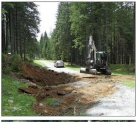
(b) Excavation material of the pipe trench with rocks of up to 1 m in diameter, in the summer of 2019.
