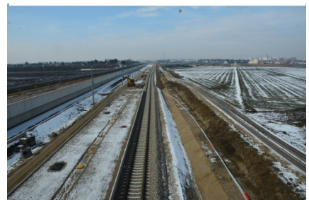
Photo 2: Almost flat gradient - challenge for stormwater management
