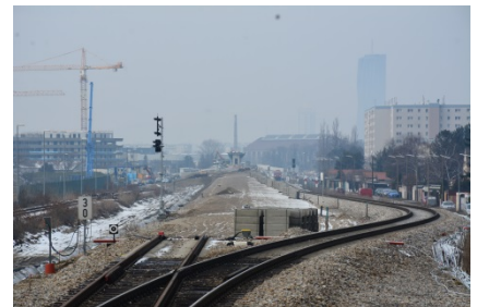
Photo 1: Construction during railway operation (diversion of track for constant operation)
