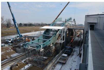
Photo 4: Construction works station Vienna Aspern North
