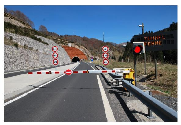
Fig. 2: Effective tunnel closure enforced by barriers, Lioran Tunnel (France) © CETU
