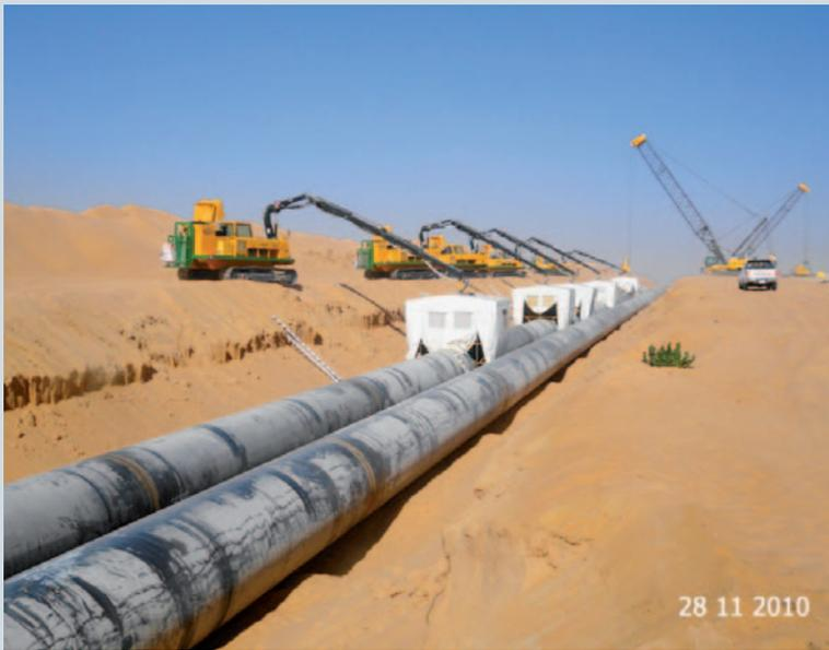
FIGURE 7: Pipeline installation works of Ras Al Khair - Riyadh
