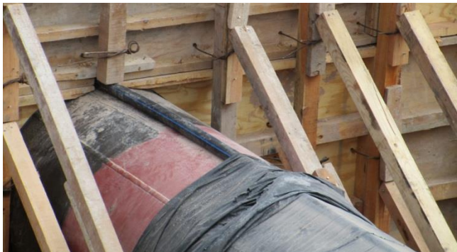
Figure 10 Position of FOC at 12 o'clock
