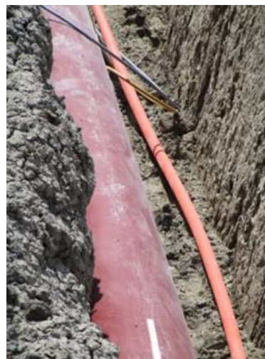
Figure 11 Pipe trench with FOC laid at 2 o'clock
