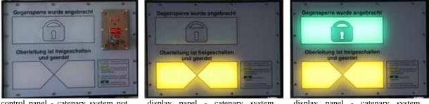
control panel - catenary system not disconnected and not grounded, and also not secured against reconnection
