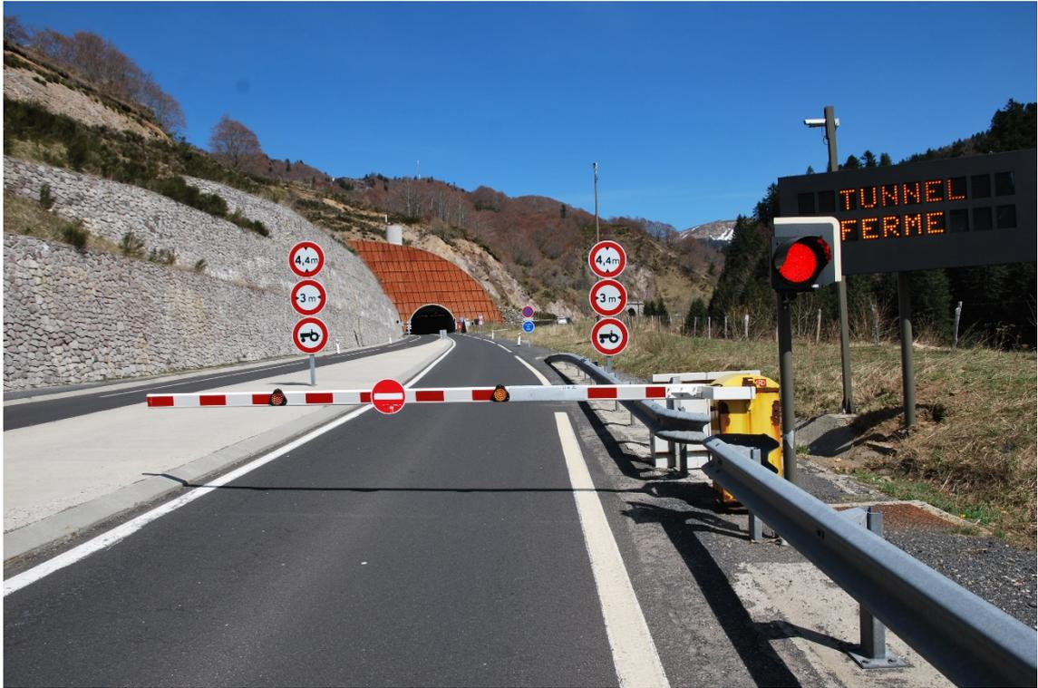
Fig. 2: Effective tunnel closure enforced by barriers, Lioran Tunnel (France) © CETU
