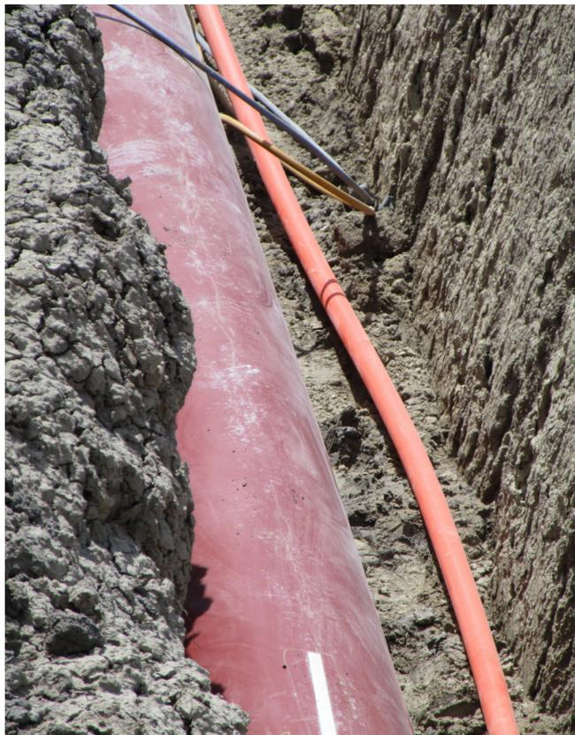
Figure 7. Pipe trench with FOC laid at 2 o'clock.
