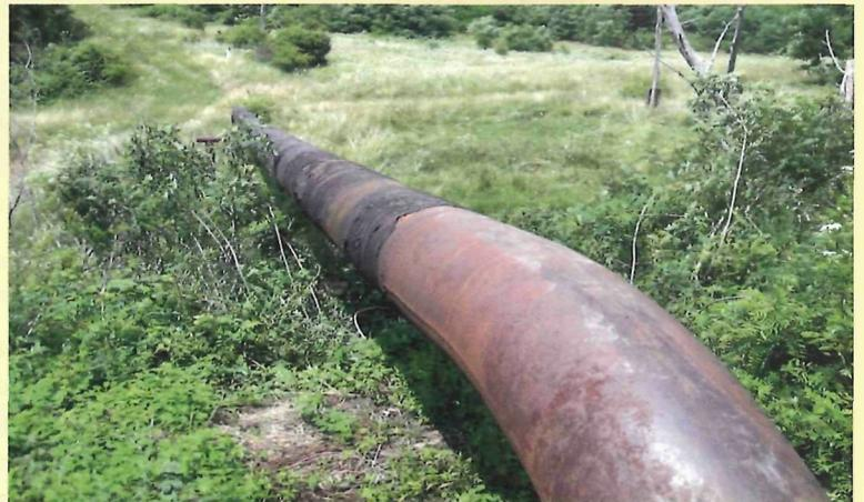
Figure 2. Ditch crossing with strange supporting and very bad coating conditions.
