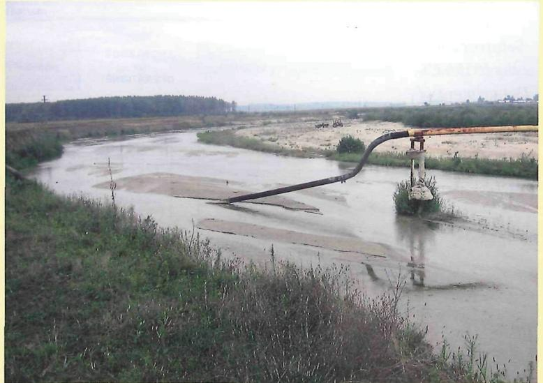
Figure 1. Above ground River crossing where the river bedding changed its position over the years.
