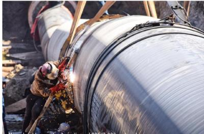
Manual welding works, 2 pipelines of 80" (2,032 mm) each
