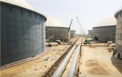
Tank farm, steel tanks: 170,000 m<sup>3</sup>, 2 pipelines of 96" (2,438 mm) each
