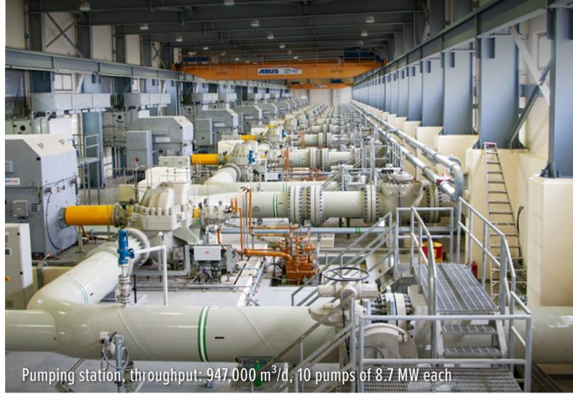
Pumping station, throughput: 947,000 m<sup>3</sup>/d, 10 pumps of 8.7 MW each
