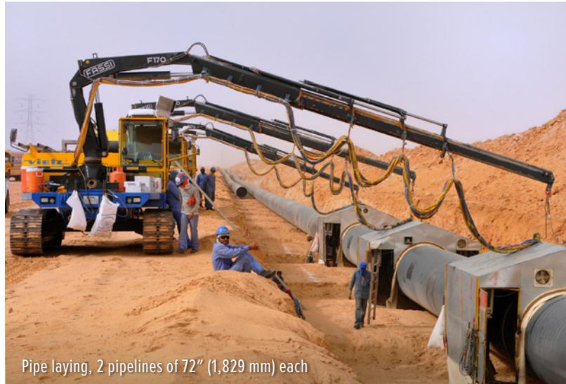
Pipe laying, 2 pipelines of 72" (1,829 mm) each
