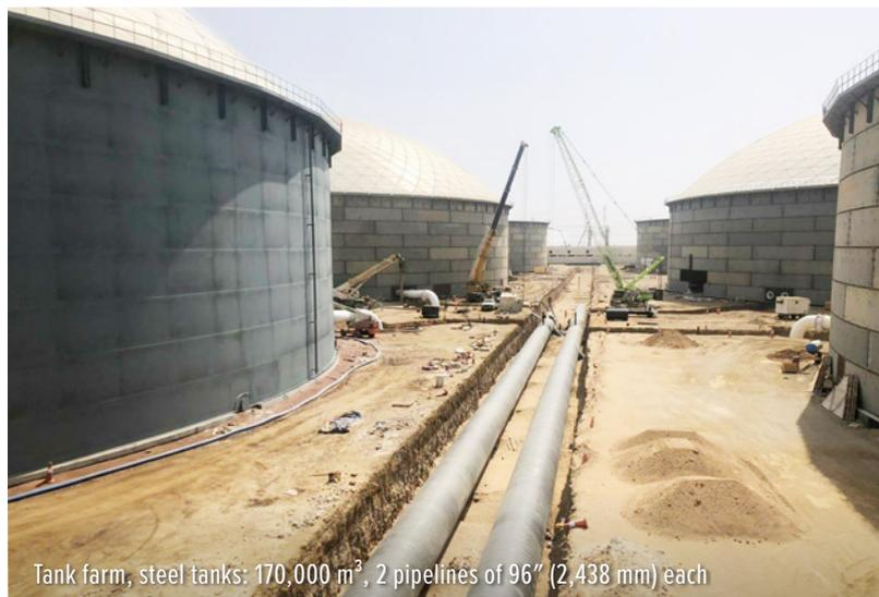
Tank farm, steel tanks: 170,000 m<sup>3</sup>, 2 pipelines of 96" (2,438 mm) each
