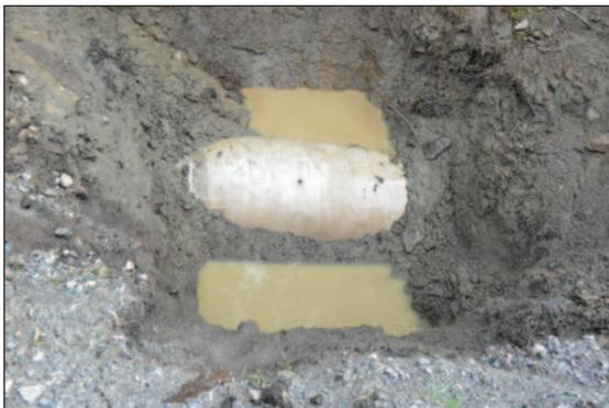
(e) Accumulation of groundwater and stormwater in the pipe trench about 48 h after rainfall event (no drainage). Same location as in Photo (d), summer of 2019.
