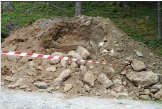
(c) Excavation/backfilling material of the pipe trench with rocks of up to 1 m in diameter, summer of 2019.
