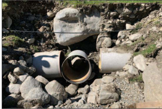
(f) Pipe damage incident no. 10 (no bedding material and unsuitable backfilling material), August 2019.
