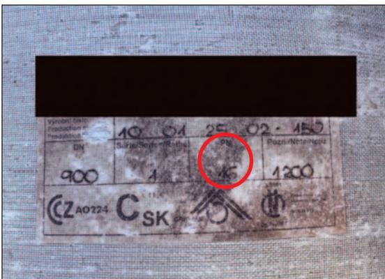
(i) Broken pipe, see photo (h) with specification sticker on pipe (pipe class PN 16 at a static pressure of 154 m water column), August 2019.
