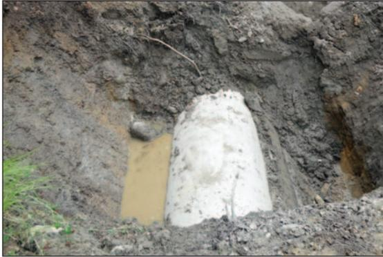
(d) Accumulation of groundwater on the embankment side after approx. 24 h in dry weather conditions (no drainage), in the summer of 2019.
