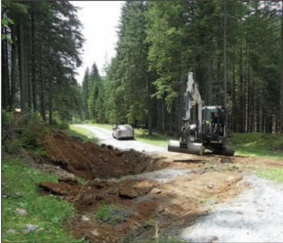
(b) Excavation material of the pipe trench with rocks of up to 1 m in diameter, in the summer of 2019.
