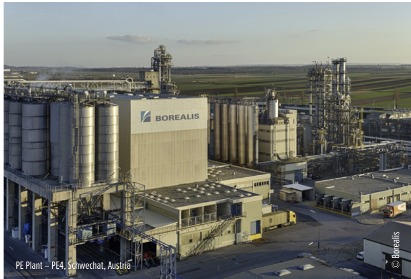
Gas-to-Urea and Polyolefin Complex
