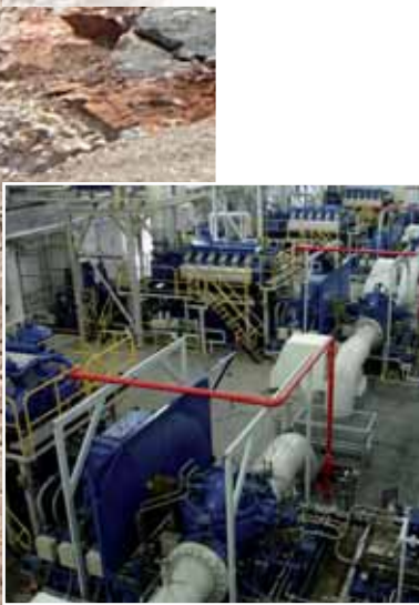
Pump station building
