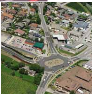
SS12 Vahrn Bypass Road, Italy
