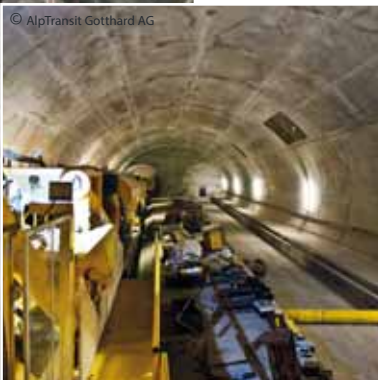
Base Tunnel at Gotthard, Switzerland
