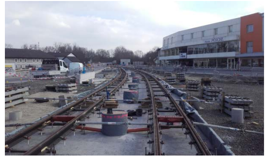
Figure 6: track during construction works © R. Schrempf
