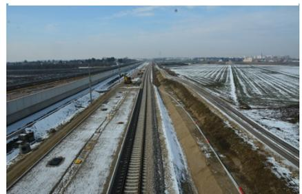
Photo 2: Almost flat gradient - challenge for stormwater management
