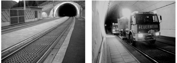
Figure 6: Access area near portal / Accessibility of tunnel by road vehicles
