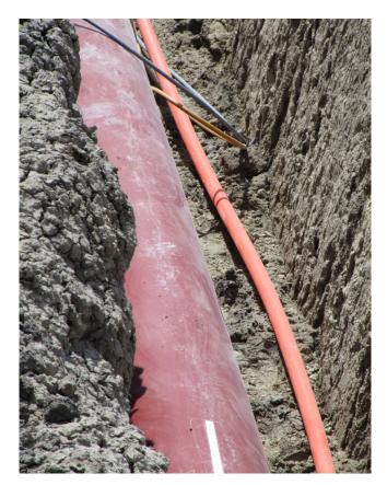
Figure 7. Pipe trench with FOC laid at 2 o'clock.
