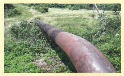
*Figure 2*. Ditch crossing with strange supporting and very bad coating conditions.
