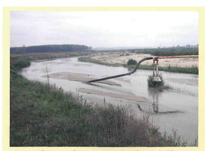
*Figure 1*. Above ground River crossing where the river bedding changed its position over the years.
