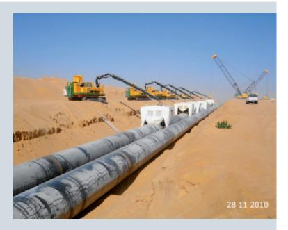
FIGURE 7: Pipeline installation works of Ras Al Khair - Riyadh
