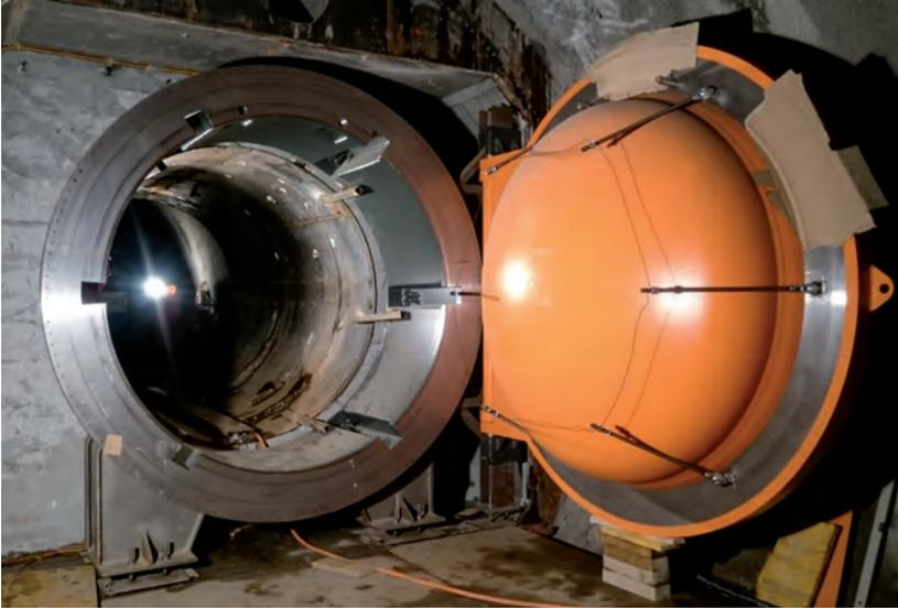
Figure 3.3.1.3.3: Rock cavern pressure vessel access door. | Source: ALACAES SA.
