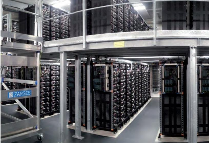
Figure 3.3.3.2.5: Interior view of the first commercial battery power station in Germany. The 5 MW lithium-ion facility has the equivalent reserve capacity potential of a conventional 50 MW turbine. | Source: WEMAG.
